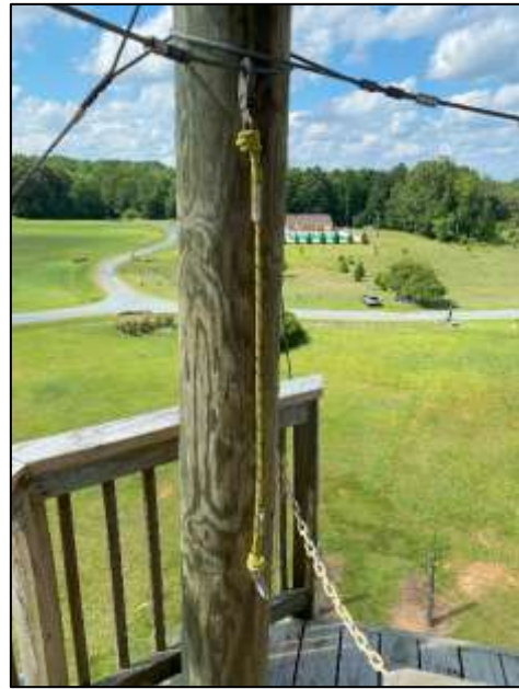
Primary participant tether for the north rappel at the Belk tower.
