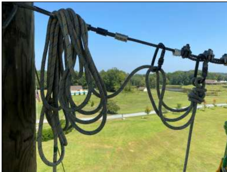
Releasable rappel on the north face of the Belk tower with the releasable line coiled and placed over the cable triangle.
