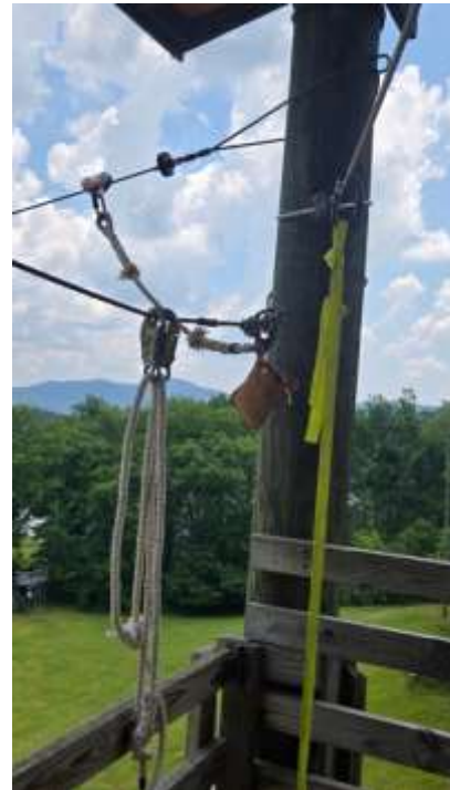
Completed zip line rigging at MSR.
